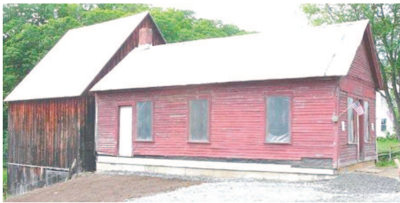
Photos of the south and north sides of the Corliss-Prescott House showing the new level roof-line, the replaced clapboards. and the new pole and pedestal on the far right.
