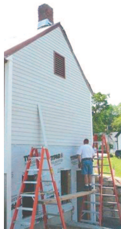
Back views of the Corliss-Prescott House in process; up on its new foundation, with new stone walls; the new clapboards on the back
