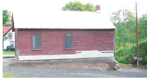
Photos of the south and north sides of the Corliss-Prescott House showing the new level roof-line, the replaced clapboards. and the new pole and pedestal on the far right.
